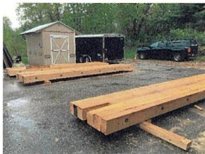
Portable laminated timber bridges
