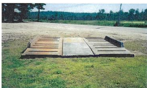
Union Hill Bridge
